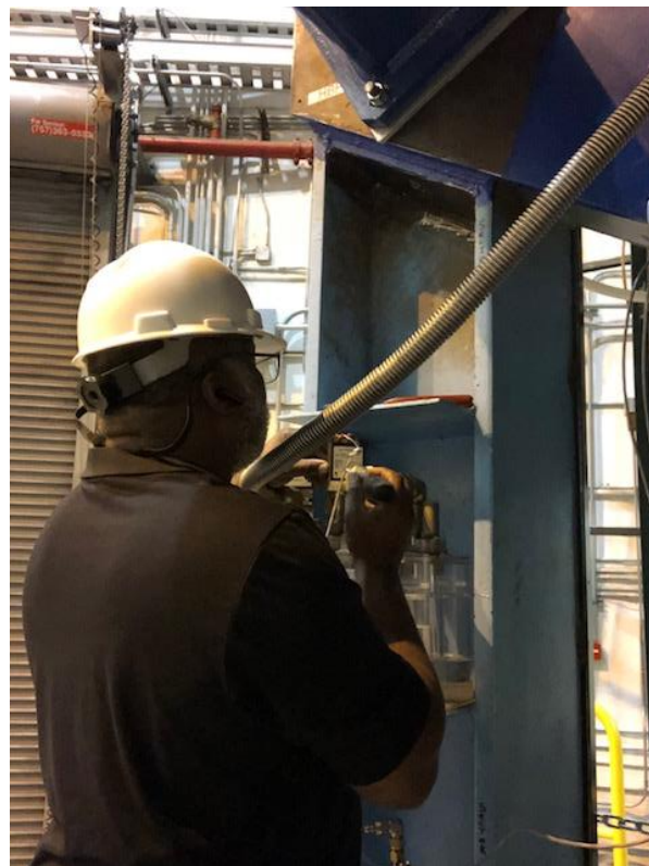
Marc McMullen connecting a Dwyer differential pressure transducer on LTCC S6 in Hall B
